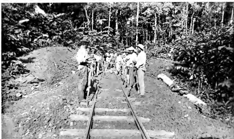
THE BALLAST GANG.
